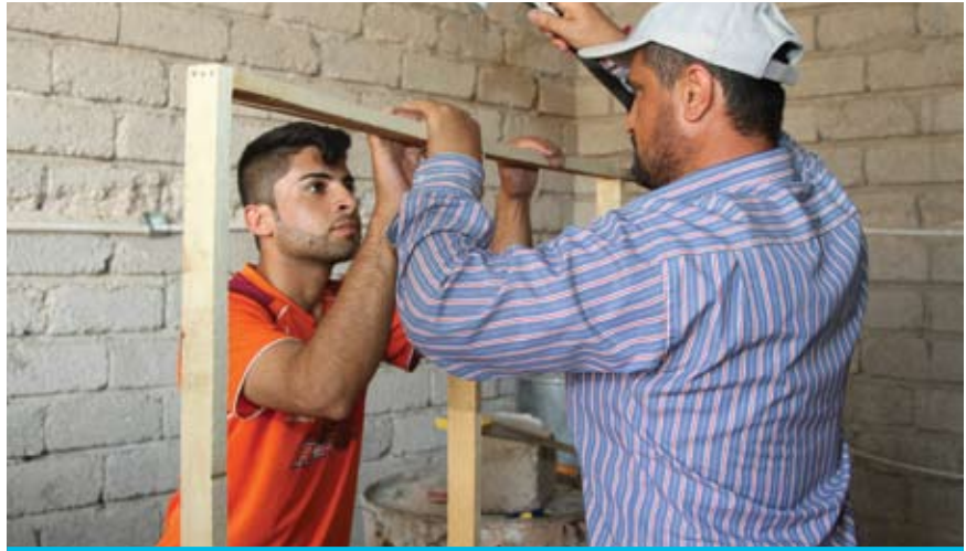
Local volunteers, most from displaced communities in northern Iraq, are trained by CRS engineers to install doors and windows in the unfinished buildings where families have sought temporary shelter. Photo by Kim Pozniak/CRS
