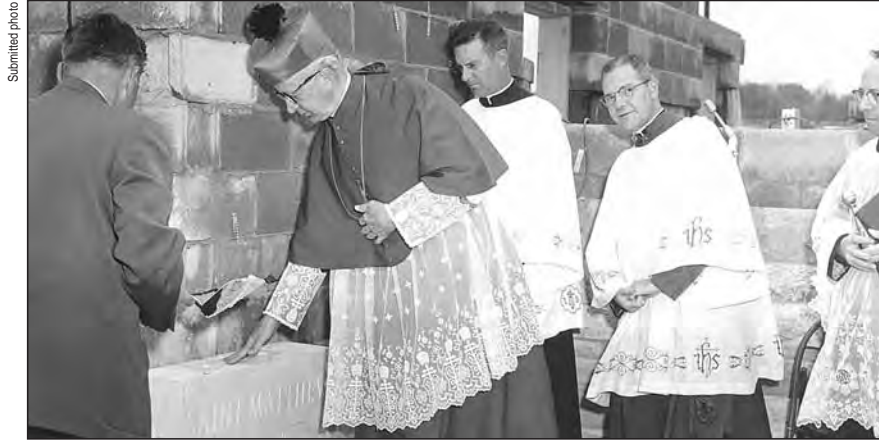
In this Archive photo, Archbishop Paul C. Schulte touches the cornerstone of St. Matthew the Apostle Church after he blessed it during the construction of the parish's facilities in 1958. Priests assisting Archbishop Schulte were, from left, Father Albert Diezeman, St. Matthew's first pastor; Msgr. Henry Hermann and Father Cyril Conen.
