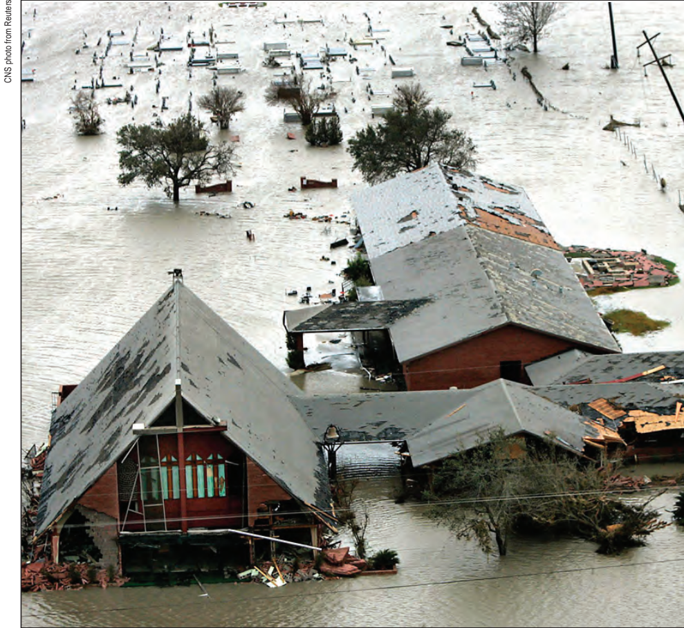
A church with a cemetery in the background is damaged in the aftermath of Hurricane Rita in Cameron, La., on Sept. 24. Hurricane Rita was the second powerful storm in less than a month that left the U.S. Gulf Coast reeling. Rita brought renewed flooding in New Orleans, widespread power outages and roads across hundreds of miles closed by debris, although damage was less than feared.
