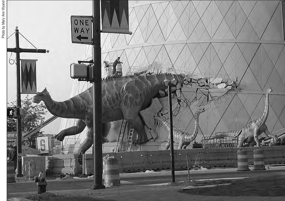
A construction worker appears to ride an alamosaur "escaping" from The Children's Museum's new Dinosphere exhibit at 30th and Illinois streets in Indianapolis. The Dinosphere opens on June 11. Indianapolis is home to the largest children's museum in the United States.
