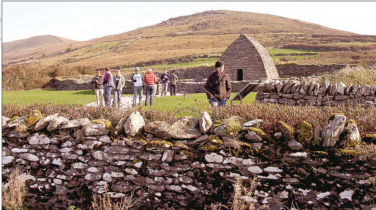
Gallarus Oratory, the first Christian church on the Emerald Isle, was built in 400 A.D., predating St. Patrick. To this day, the small dry-masonry structure facing the Atlantic Ocean is waterproof.
