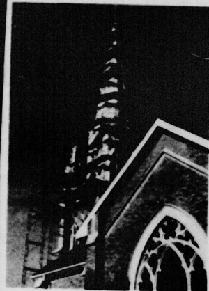
A STEEP PROJECT—In preparation for its sesquicentennial celebration this year, St. Vincent de Paul of Shelby County restored its church tower and steeple last fall. The lower, unusually constructed for its 1834-35 vintage, is made of concrete placed on a steel frame. (Photo by Bette Lux)
