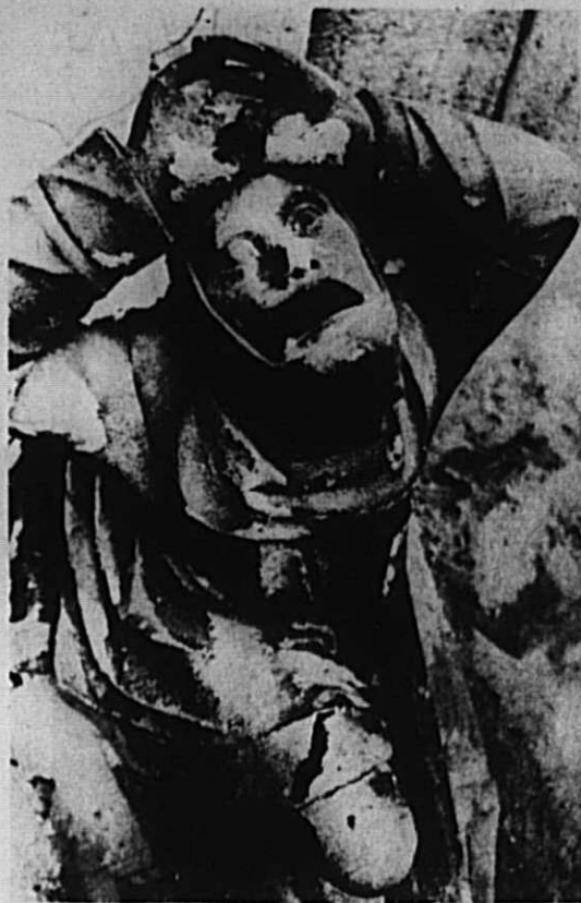
THREATENED BY POLLUTION —The twin-spired cathedral in Cologne, largest of all German churches and one of the chief monuments of Gothic architecture in Europe, is seriously threatened by air pollution. As the statuette at left illustrates, the richly ornamented cathedral is threatened by corrosion. The white patches are evidence of chemicals from Cologne's polluted atmosphere turning the solid sandstone into powdery white gypsum. According to a recent report, the cathedral stone work has been decaying so rapidly as a result of industrial
