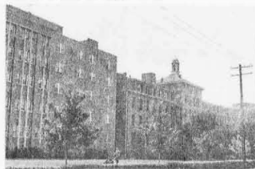
ST. FRANCIS HOSPITAL
